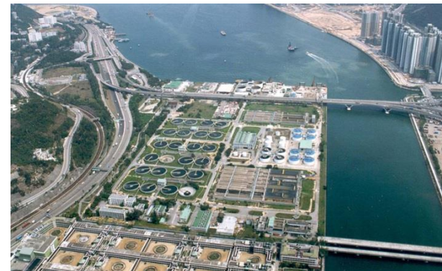
Water / Wastewater Treatment Facilities
