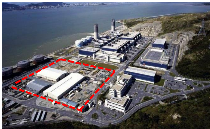
New Combined-Cycle Gas Turbine
