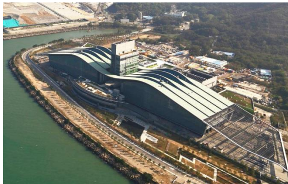
Sludge / Waste Treatment Facilities
